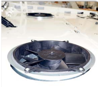
Axial fan of the filter unit (exhaust air)
